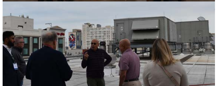
Into and above the guts of PACC Mechanical Systems
